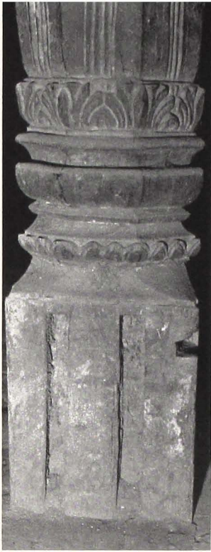
106 The Third Floor, Vestiges of a Post
