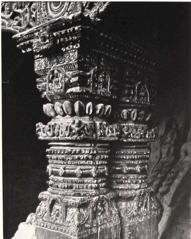
91 Mani Keshav Narayan Chok, South Wing, Pillars of Dalan
