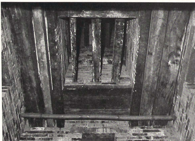
80 Agan Mandir, Structure view from the First Floor (M2-13)
