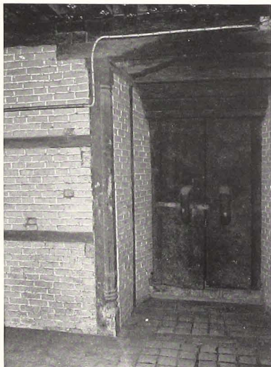
105 The Third Floor, South Room, Post
