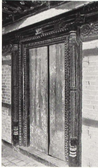
107 The Fourth Floor, North Room, Entrance to South Room
