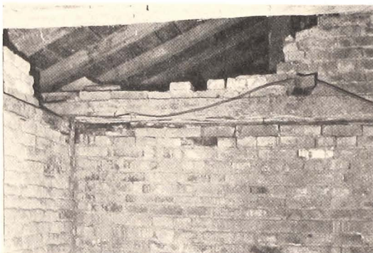
Fig. 1-1-17 South Wall of the Room 'M2-2'.
