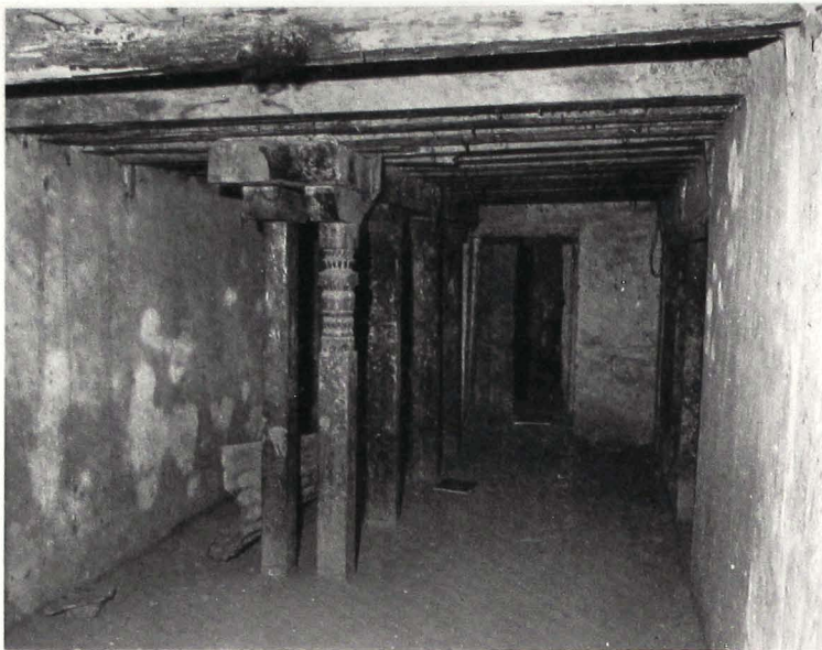
78 Mul Chok, South Wing, the First Floor (M2-13)
