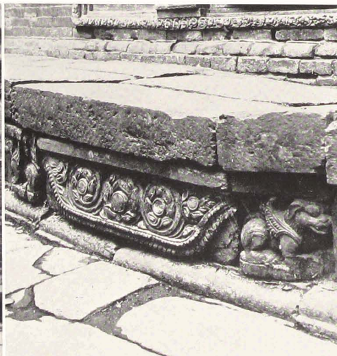
54 Sundari Chok, South Wing, Stone Carving of Foundation Bed
