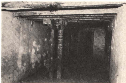
Fig. 1-1-23 The Room M 2-13 Facing West.
