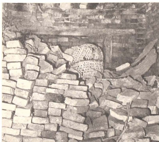
Fig. 1-1-11 North Wall of the Room 'M1-4'.
