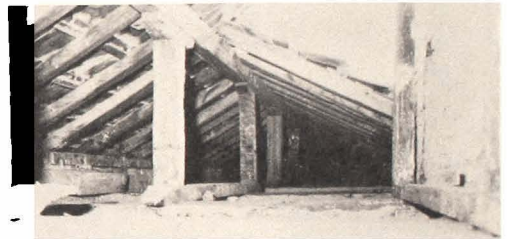
Fig. 1-1-11 Roof Structure of the Room 'S3-2'.
