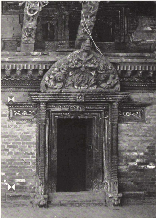
76 Mul Chok, West Wing, Entrance (1W-22)
