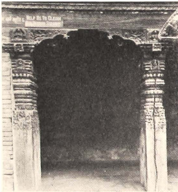
Fig. 2-3-1 Thick Pillar of East Wing, Sundari Chok.
