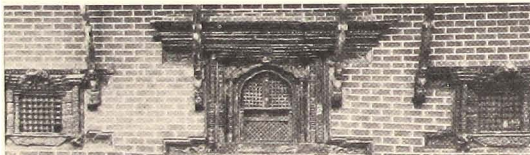
Fig. 2-4-16 Window '2W-3', Mani Keshav Narayan Chok.
